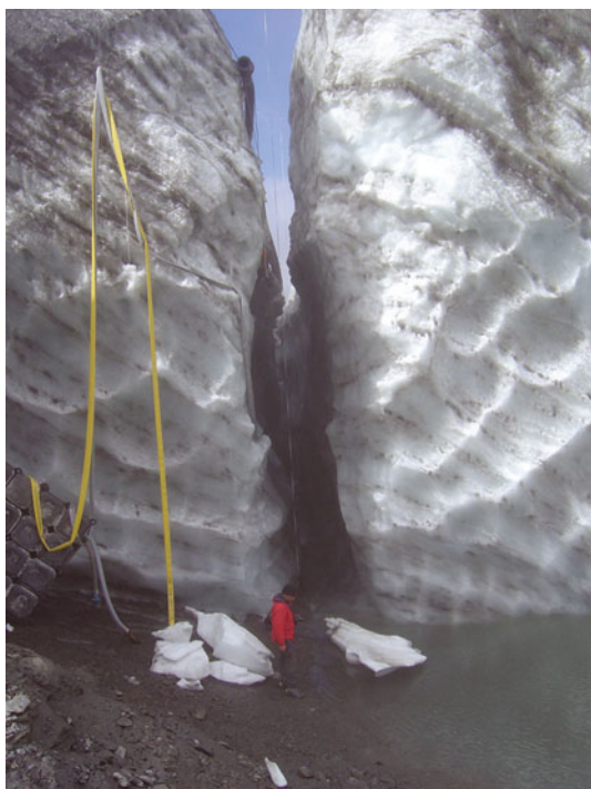
Fig. 2. Channel dug through the ice during drainage. The top 6 m were dug artificially using explosives, then the water overflowed through the ice breach and dug the channel naturally. (Photograph by C. Vincent.)
