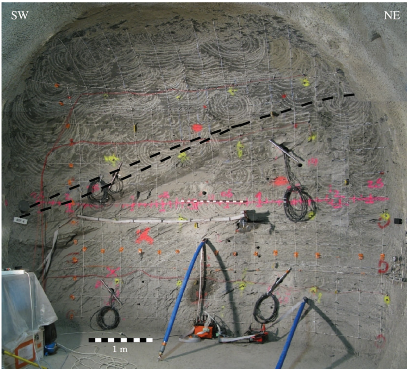
Figure 2. General view of the geophysical monitoring system installed on the Ga04 side of the EZ-G section. A tectonic fracture (SW dipping fault N 120–20°) well visible on the face is marked by a black dashed line. The white mesh has a mean side of 30 cm and represents the mesh formed by horizontal and vertical lines of the array of 700 electrodes installed to perform a detailed electrical tomography of the EDZ-04. The distance between the electrodes along the lines is 15 cm.
