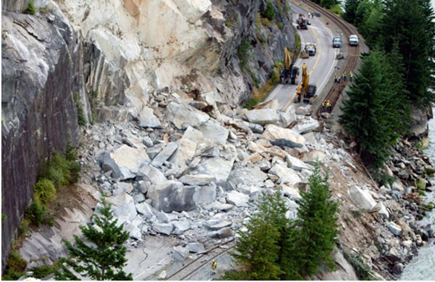
Fig. 1. Rockfall on Sea to Sky highway (B.C.). Note the jointed structure of the source area (Canadian Press photos).
