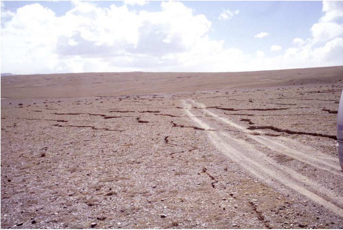
Figure 5. Cracks along the road from Kusai Hai to the Kunlun pass. At this point, the road is several kilometers from the fault. The cracks were not mapped and their orientation was not specifically measured, but was close to the orientation shown in Figure 4. The cracking is consistent either with extension or with compression and inelastic yielding followed by tensional failure when the compression was relaxed.
