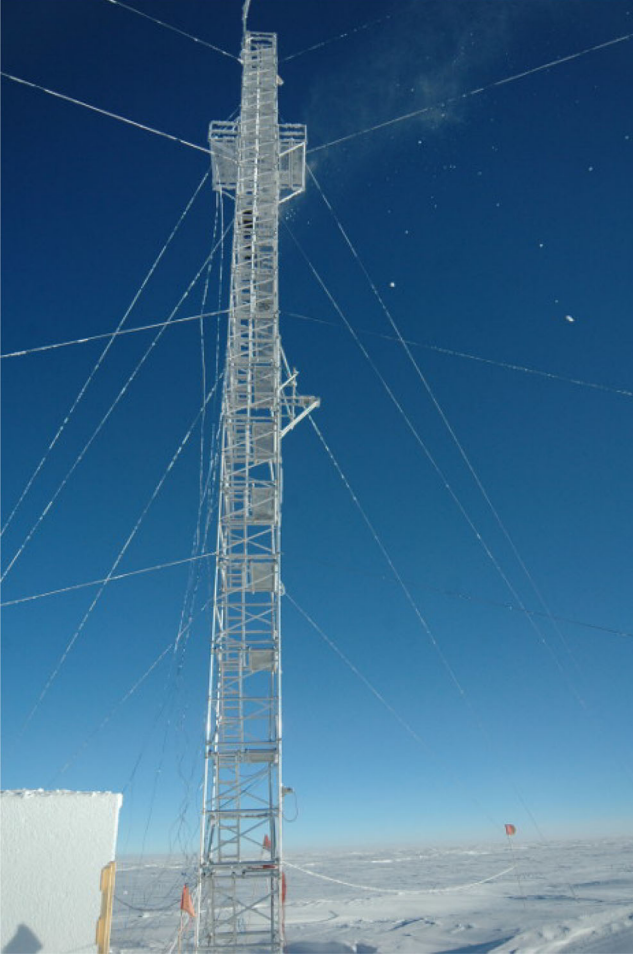
Figure 1. The 45 m tower at Dome C. Computers and electronic equipments are located in the shelter at the foot of the tower.
