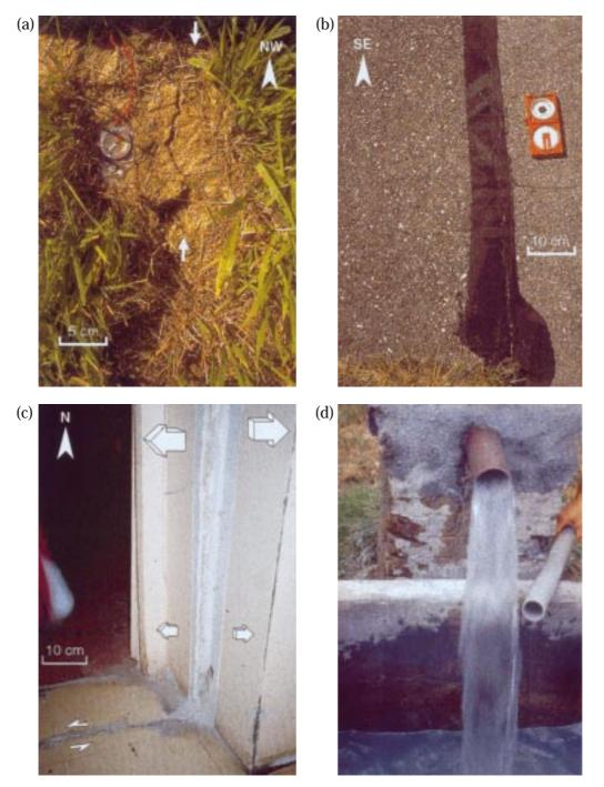
Figure 11. Ground cracks (a) a few metres west of and (b) on the runway of the Annecy–Meythet airport; see Fig. 7 (RC) for location. (c) Leftlateral strike-slip displacement at the Chaumontet warehouse; see Fig. 7 (CW) for location. (d) Output increase at Bromines spring, with old pipe and new pipe; see Fig. 7 (BS) for location.
