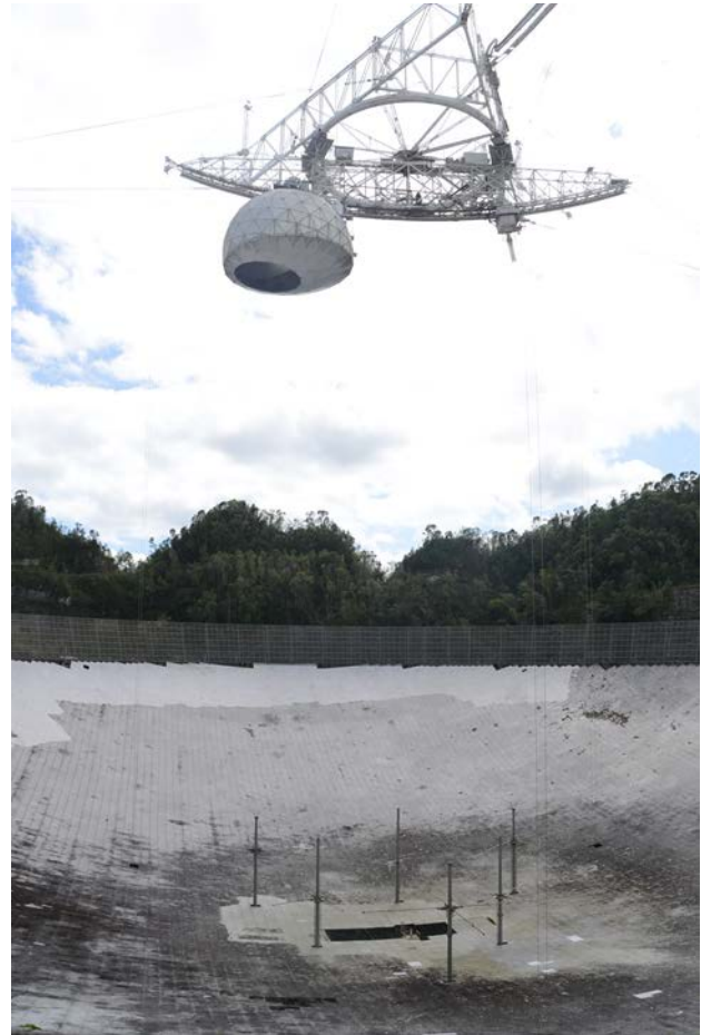
Figure 2.4. The HF antennas in the center of the Arecibo reflector. A wire mesh HF subreflector, not easily resolvable here, hangs under the platform on top of the HF antenna. The sub-reflector altitude is adjusted according to the selected HF frequency.
