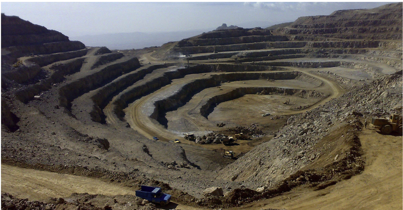
Figure 2. View of the Angouran open pit; the brown color correspond to the non-sulfide ore. Host rock of the non-sulfide ore is marble.
