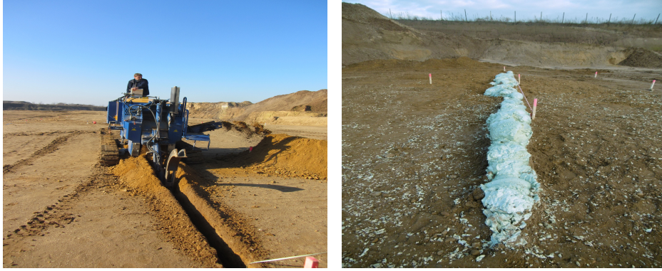
Figure 4: Wheel trench device and injection of geofoam
