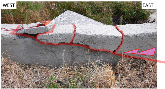
Figure 6. Field photograph of compressive features affecting recent concrete dykes after the Hengchun earthquake (26 December 2006, M_L = 7.0 ); see location in Fig. 1 near the Fang-Shan village ( 22.26^\circ N, 120.66^\circ E). The red compass gives the scale of the outcropping deformation (20 cm). The thrust is associated with three back thrusts, highlighting a small pop-up (below the compass). The red arrow reveals the thrusting component that affects the new concrete dykes.
