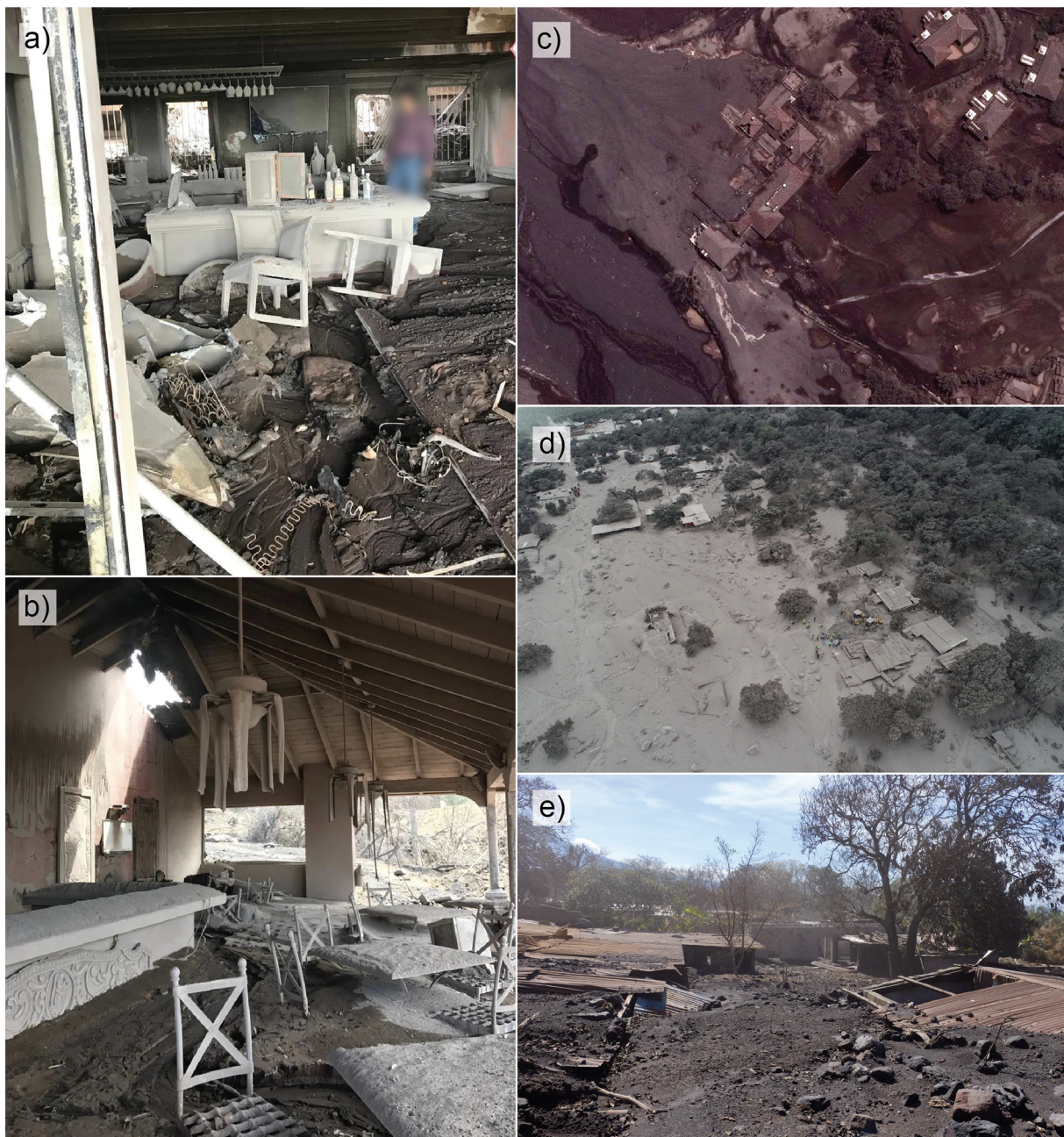
Fig. 9. a) inside of La Reunión clubhouse building showing effect of LEDS (ash-covered bottles on counter) and post-eruption lahars (knocked over chairs) (22 June 2018), b) inside of clubhouse building showing overflow deposits to chair height, LEDS deposits of a few centimetres on tables, isolated fire damage to roof, and ceiling fan melted due to radiant heat from overflow deposits (22 June 2018); c) Digital Globe satellite imagery of La Reunión golf resort (acquired three days after impact on 6 June 2018) showing partially inundated clubhouse building. Different shade of grey between left and right side of the buildings shows deposition areas of dense overflow flows (L) which were stopped by structures and LEDS (R) which were able to flow past (adapted from imagery provided by Maxar Technologies under CC BY-NC 4.0); d) aerial photo of San Miguel Los Lotes, facing south, showing fully destroyed northern end of town (bottom of frame) with large boulders, contrasted with mostly undamaged buildings at the south end of town (top left of frame) (AP, 5 June 2018), e) buried buildings in the town of San Miguel Los Lotes showing minimal structural damage and deposits surrounding and on top of buildings (P. J. Baxter, 25 June 2018).
