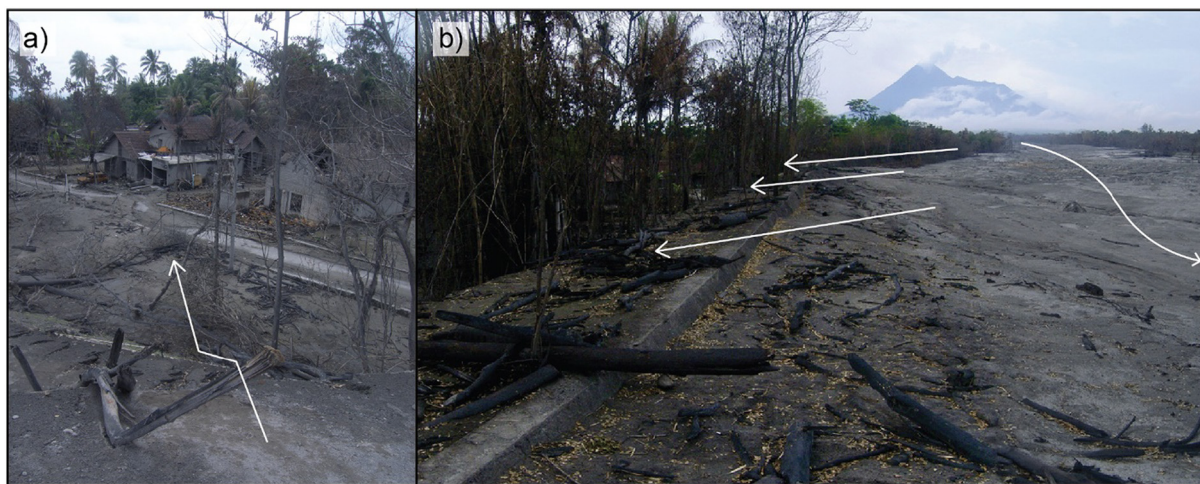
Fig. 4. Photos taken from the top of the concrete levee bordering the Gendol and adjacent to Bronggang village: a) Looking southwest down the levee and in the direction of LEDS spillover into Bronggang village; b) Looking north up the infilled Gendol channel with LEDS and small flow overspill into Bronggang to the left of the image. Charred tree branches and embers (firebrands) that were carried within the PDC can be seen on top of and within deposits in the channel and in the village. Photos taken by S.F. Jenkins 25 days after impact on 30 November 2010.
