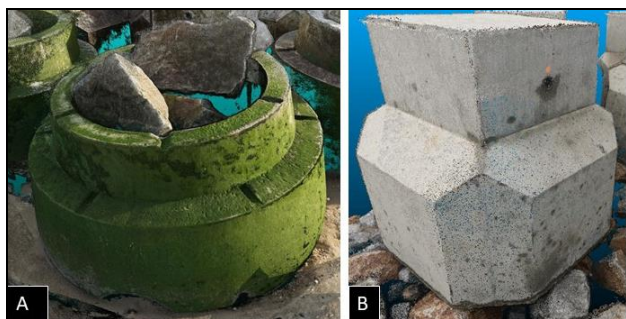
Figure 1. A: Accroberm™ II (2.24 m diameter); B: 'double cube' unit (1.3 m nominal diameter)
