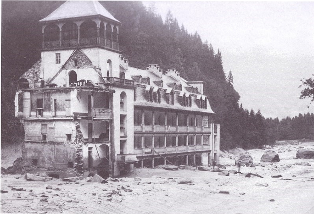
Figure A1. The wiped-out thermal bath of Saint-Gervais-les-Bains after the debris flow of the 12 July 1892 (thermal bath establishment of Saint-Gervais, via https://www.thermes-saint-gervais.com/ , last access: 24 February 2022).
