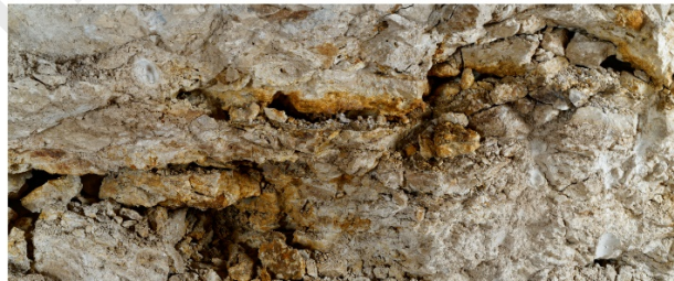
c) Fractured limestone rock (depth=16 m)
